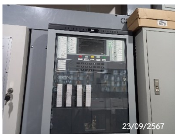
Fire Alarm Control Panel
